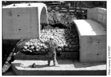
A pre-fabricated culvert is shown being installed over field stones in the Conference House Park Bluebelt.
