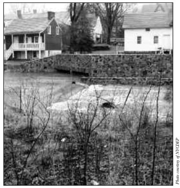
The weir of the historic Mill Pond was rebuilt to safely convey flows from the storm sewer network that was constructed in the Richmond Creek watershed.
