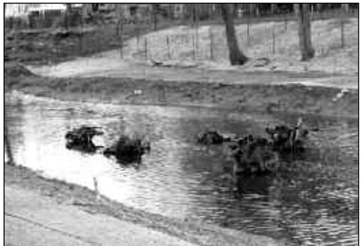
Root wads shown here were driven into a pond bottom for wildlife habitat. The wads were submerged as the restored pond filled with water.
